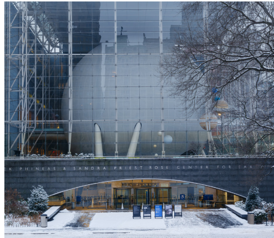
Rose Center for Earth and Space Located on 81st Street near Central Park West
