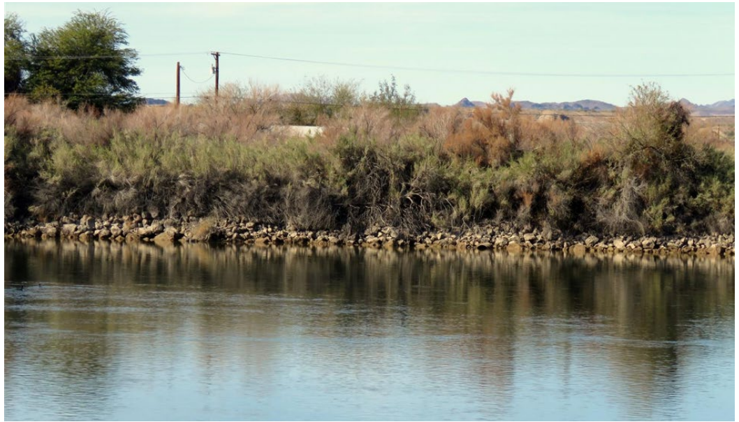
Figure 2. Rip-rap along the banks of the Colorado River. Photo credit: L. Harter.
