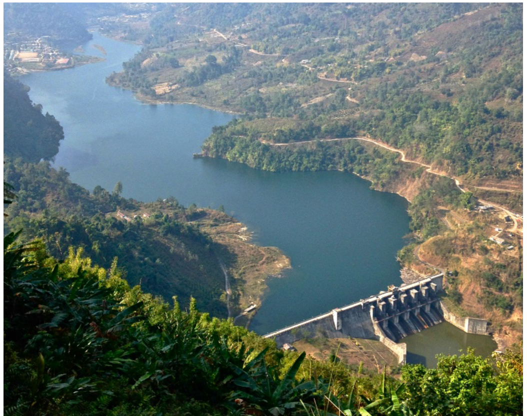
Figure 4: The Ranganadi Hydroelectric Project (405 MW) in Arunachal Pradesh (photo credit: Costanza Rampini, 2014).
